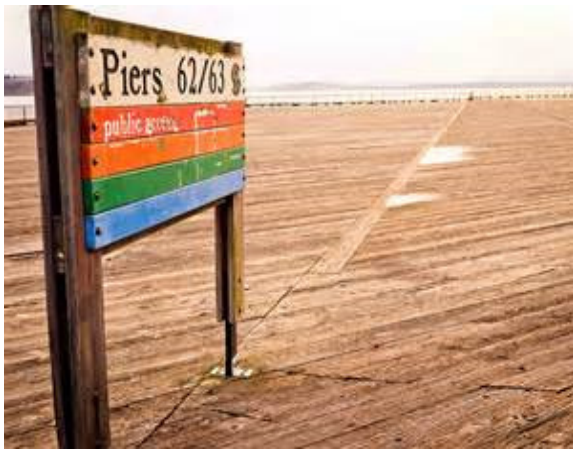
Figures 2 and 3: Pier 62/63 Existing Conditions
